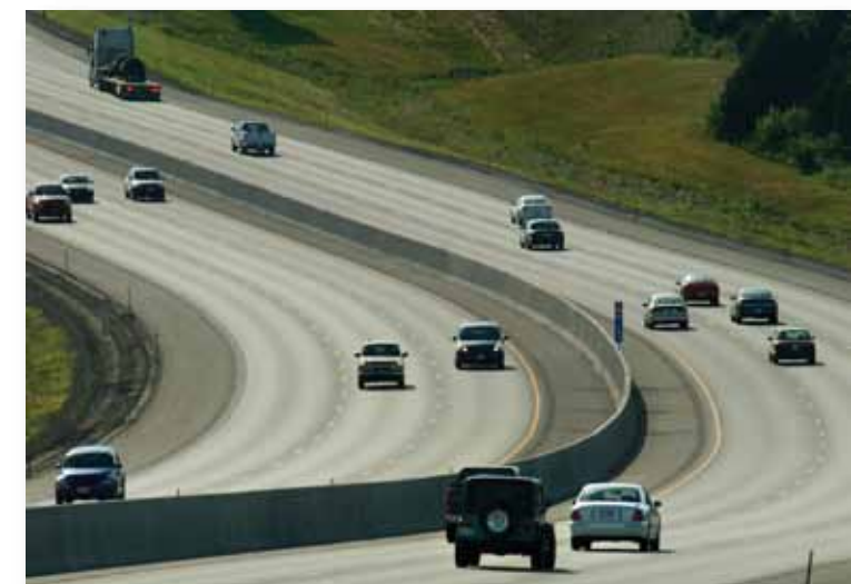
Six-lane section recently widened along I-70.
