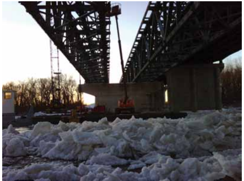
KRB - We are getting ready for tomorrow's blast. The picture shows our barge work platform where ice pack is starting to move in.
